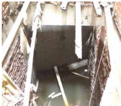
Water collection area in a construction site
